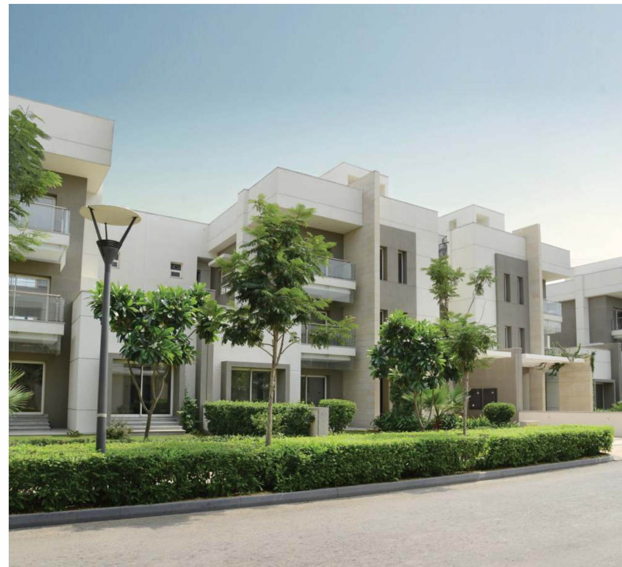
ACTUAL IMAGE OF DUPLEX VILLA, BLOCK E
