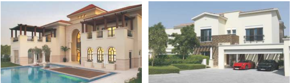
SOBHA District One, MBR City, Dubai
