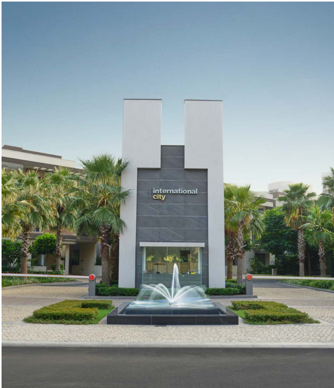
ACTUAL IMAGE OF THE BLOCK B ENTRANCE
